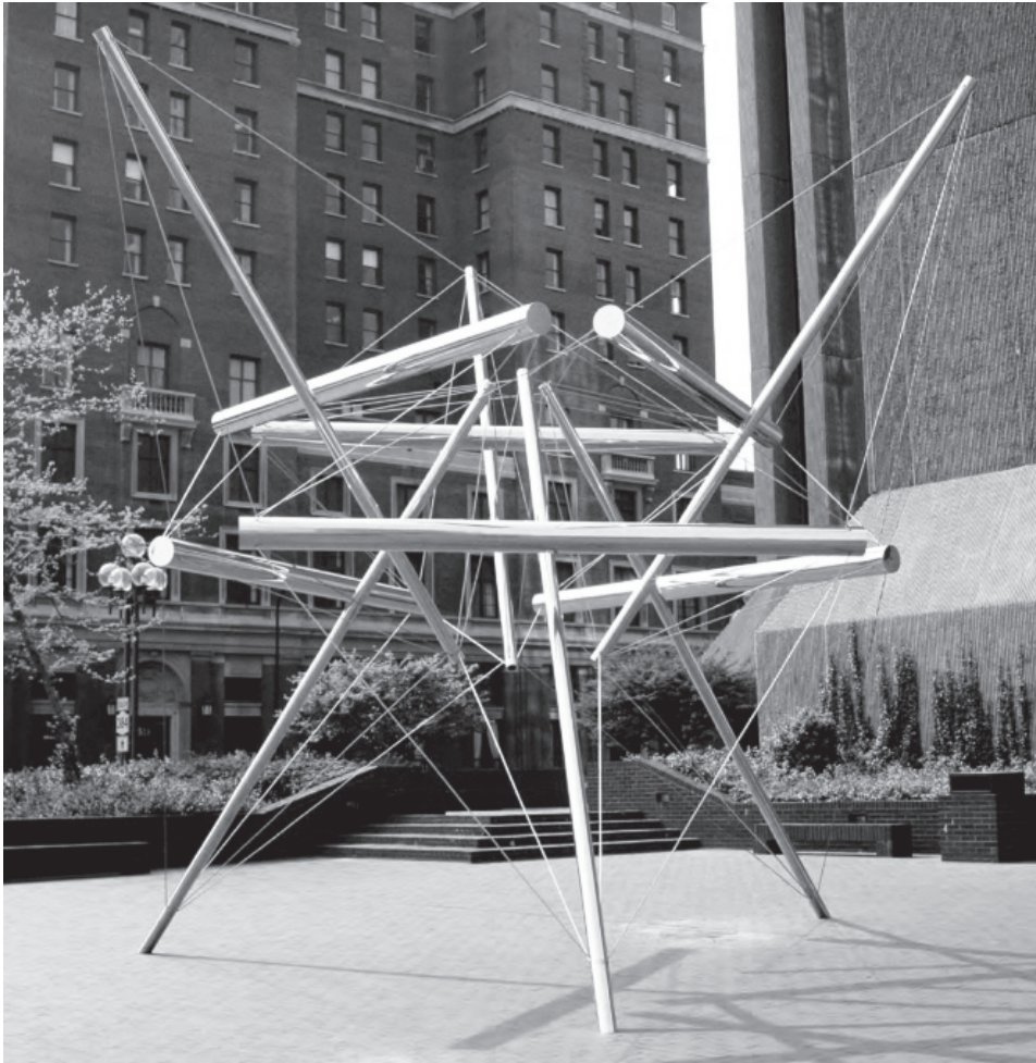
Figure I.8.2 A tensegrity structure on a plaza in Buffalo, NY, USA. (Credit: Snelson & Heartney, n.d.)
